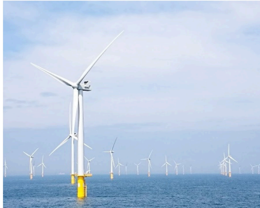
Figure 1. The Nobelwind offshore wind farm was inaugurated in May 2017 and uses 3.3MW wind turbines on monopile foundations
