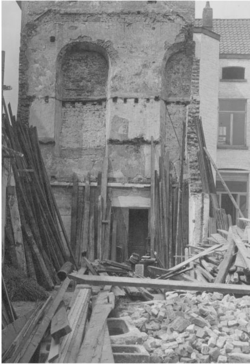
Figure 5. Sorting materials (brick, timber, blue stone) at the demolition site of Chartreux Chapel in 1905. Rue des Fabriques 1 in Brussels. Collection Comité d'Etudes du Vieux Bruxelles © KIK-IRPA Brussels.
