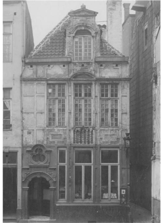
Figure 6. The facade of the Gouden Huyve situated in Rue de l'Etuve 13 was carefully dismantled in the 1920s and reconstructed in 1929 next to Sint-Nicolas Church. Collection Comité d'Etudes du Vieux Bruxelles . © KIK-IRPA Brussels.
