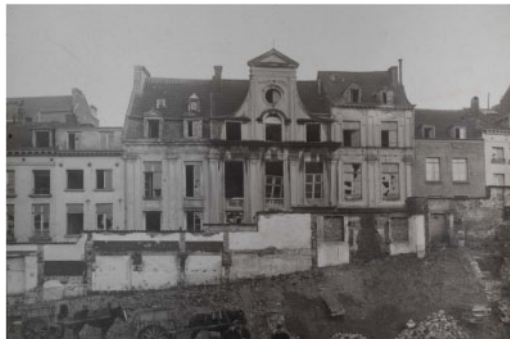
Figure 4. Window frames are taken out of the buildings before demolishing the houses on Rue Montagne de Sion. Collection Comité d'Etudes du Vieux Bruxelles © Bibliothèque artistique, ArBA.
