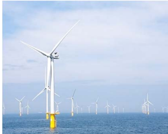
Figure 1. The Nobelwind offshore wind farm was inaugurated in May 2017 and uses 3.3MW wind turbines on monopile foundations
